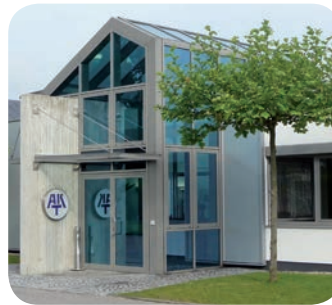
PLANT BOTTROP IDLERS AND CONVEYOR BELT ROLLERS
